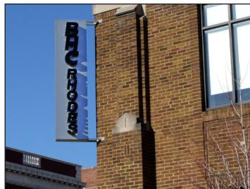
**Projecting Signs** can complement the architectural detailing on older buildings. Contrasting materials like metal and cut letters can enhance this effect.
